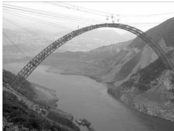
Fig.4: Installation of arch ribs
