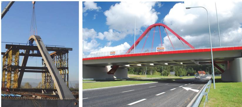
Figure 5: Assembly of the arch and view of completed viaduct in Jelenia Góra
