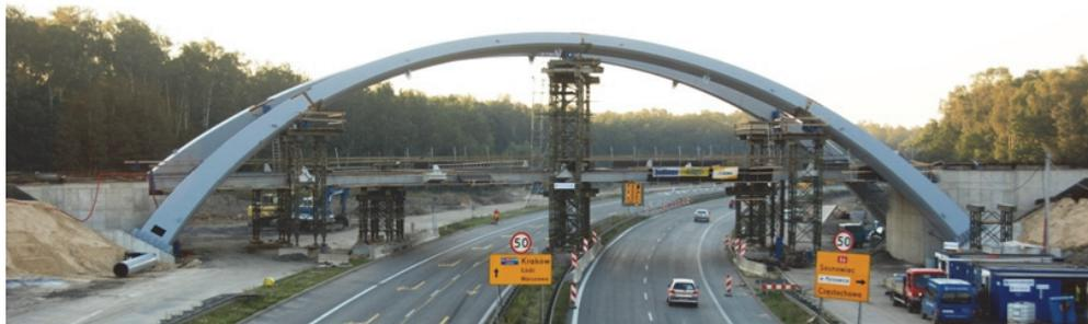
Figure 9: Overall view of one of the arch viaducts in the “Murckowska” interchange in Katowice during construction [4]
