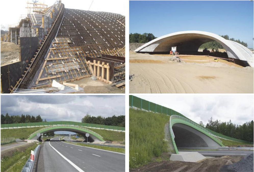
Figure 7: Green viaduct – photos of construction stages and views of completed structure
