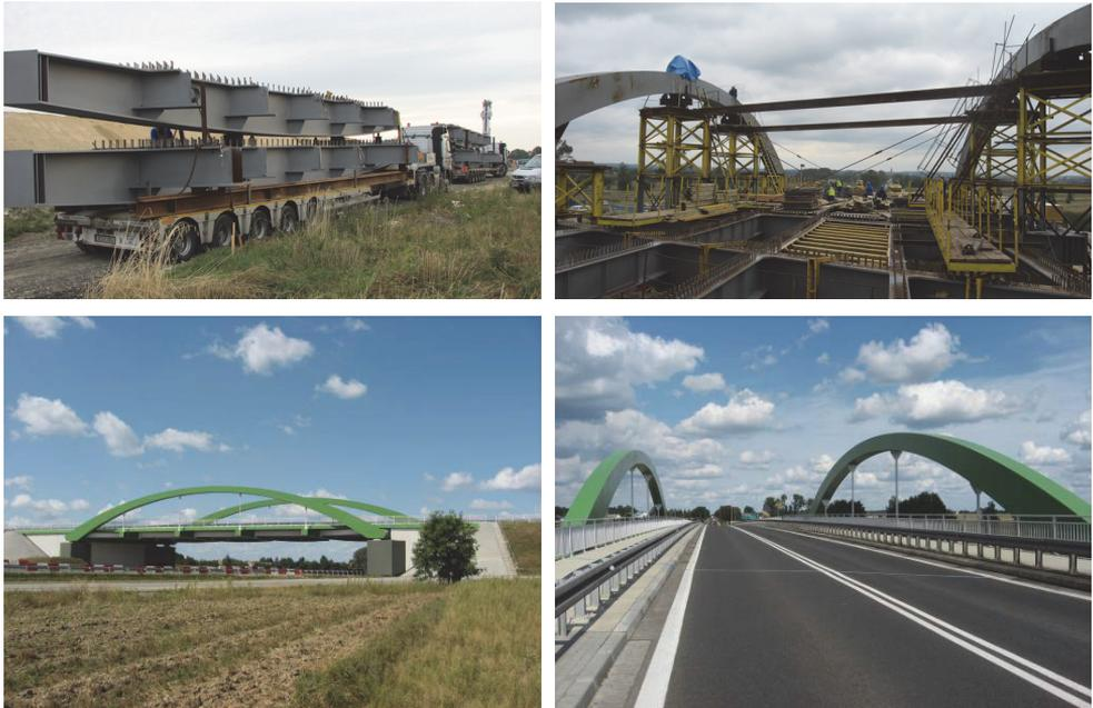
Figure 3: Views of the viaduct in Stryków during construction (photo: P. Pilczuk, VISTAL Gdynia S.A.) and view of completed structure
