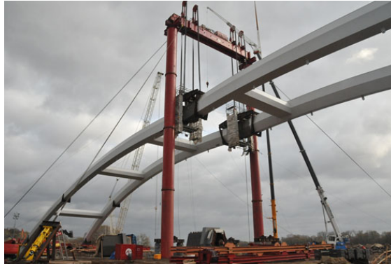
Fig. 9. Lifting tower – arch head joint.
