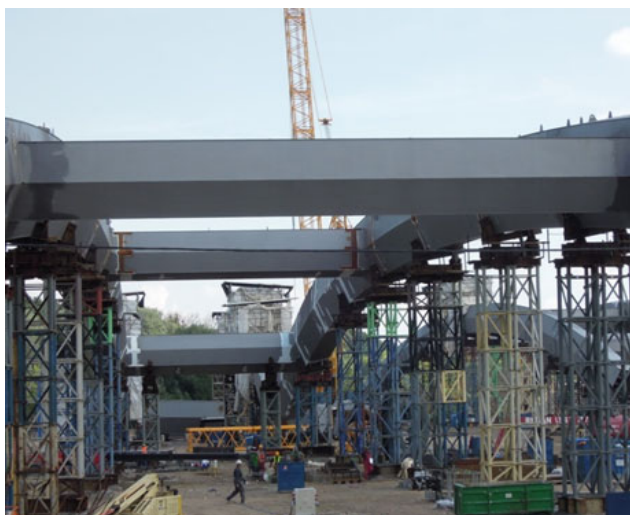
Fig. 7. Assembling half-parts of arch on temporary support.
