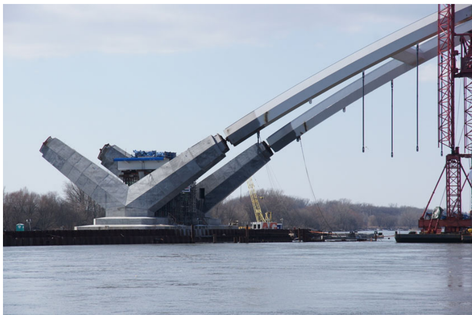
Fig. 14. Placed on support first arch.
