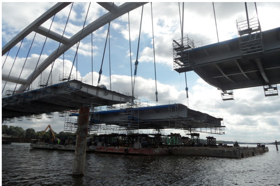
Fig. 14. Lifting deck segment.
