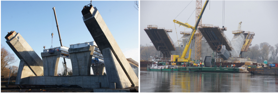
Fig. 4. Arch beds of middle support (left) and arch beds of side support (right).
