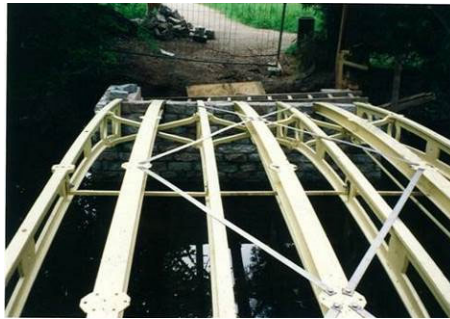
Fig. 20. Four original cast iron arches and three later added arched beams [8].
