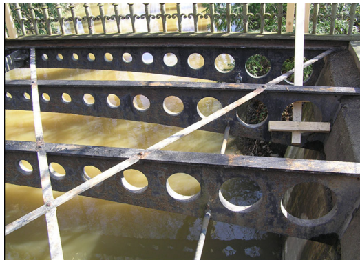
Fig. 9. Bridge structure during rehabilitation works in 2014.
