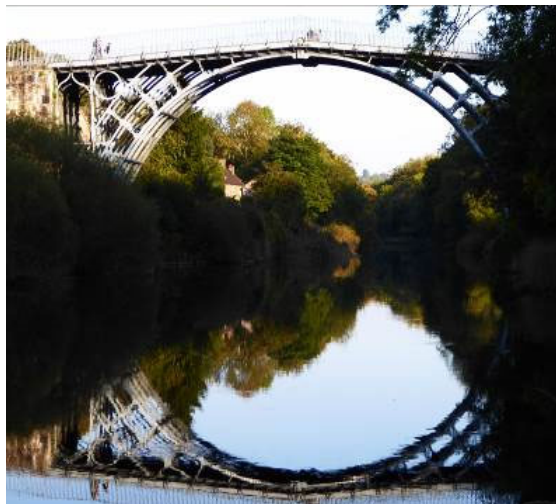
Fig. 1. Iron bridge in the iron gorge.
