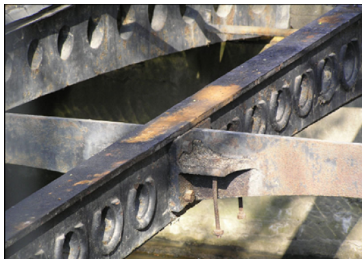
Fig. 10. Transverse stabilization in the vertex of the arch.
