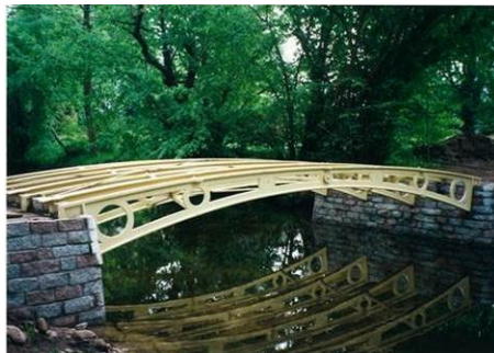
Fig. 21. Schwerin castle garden bridge during rehabilitation [8].
