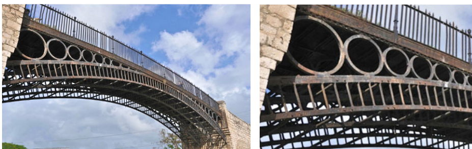
Fig. 8. Earliest cast iron arch bridge (left) in the Western Hemisphere in Spanish town, Jamaica, with corroded surface (right), [6], Photo (2010): by courtesy J. Pheasant.
