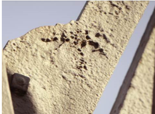
Fig. 2. Raw upper surface of the arches cast in open sand moulds.
