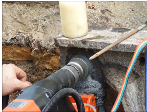
Fig. 13. Core drilling at Bad Muskau cast iron arch [7].
