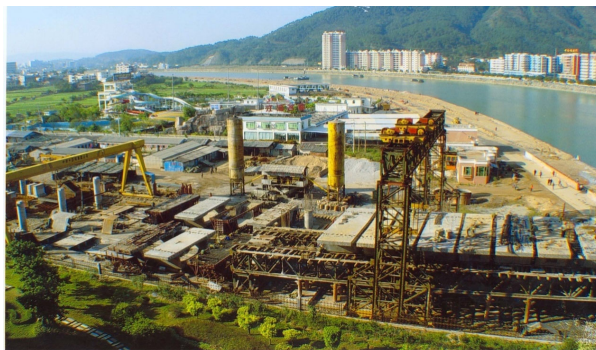
Fig. 5. Box girder casting yard and assemble platform.
