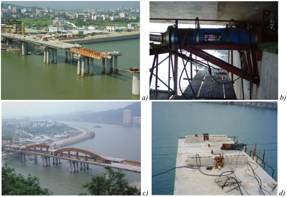
Fig. 7. Incremental launching process of continuous box beam: a) photo of incremental launching, b) 100 t continuous jack, c) construction of steel tube main arch, d) slide equipment.
