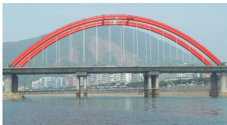
Fig. 9. Construction of beam arch combination bridge.
