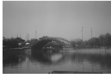
Fig.13: False timber arch Bridge
