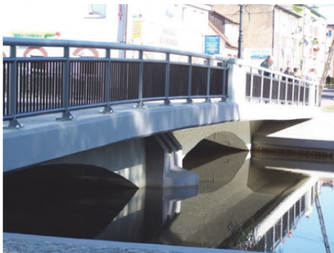
Figure 7: The bridge at opening (2009)
