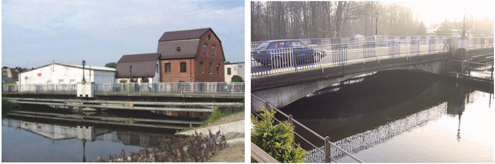
Figure 2: General views of the bridge with the historic hydroelectricity plant
