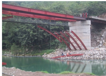
Fig. 9. The girders are used as a travel crane and with the help of a trolley pole the rest of the arch ring pieces are moved through the span.
