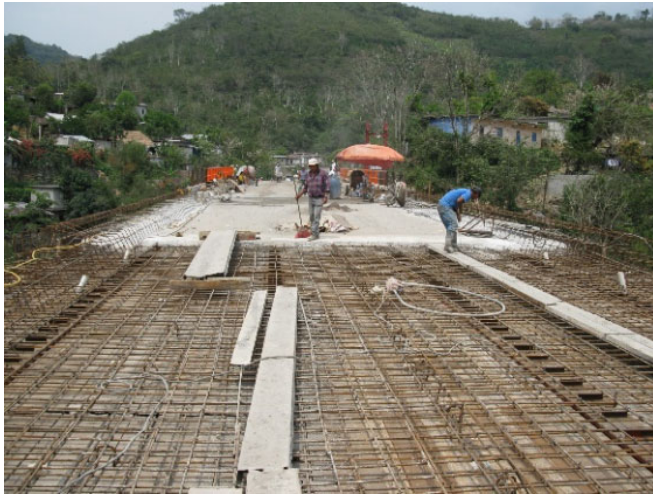
Fig. 11. Final stage, the concrete slab.
