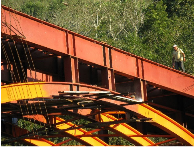
Fig. 10. The camber is counteracted using hydraulic jacks, the positioning the spandrel columns.
