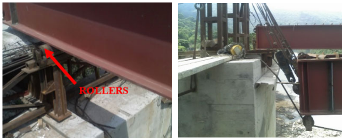
Fig. 8. The girders are located over rollers that allow the movement, the girder are pulled till they reach the pile with the truss towers.
