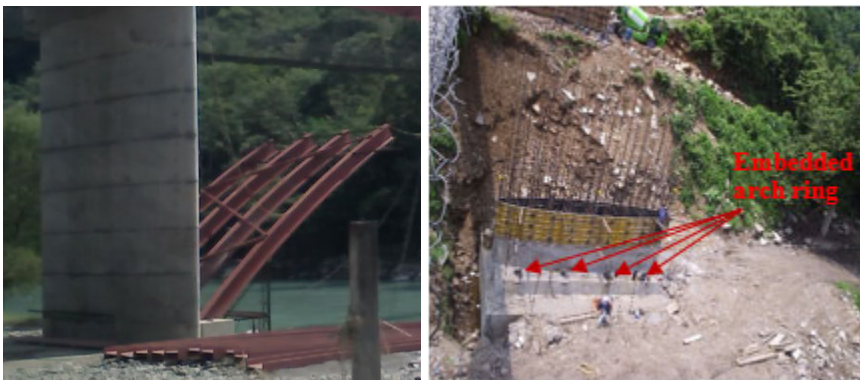
Fig. 3. Start of the arch ring embedded on the foundation.
