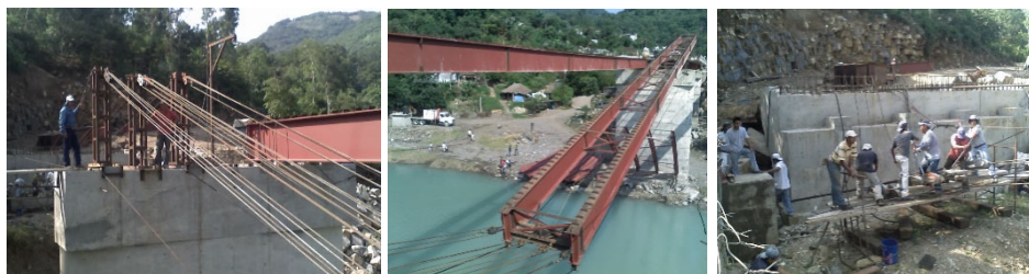
Fig. 7. Truss towers with a pulley, one end of the cable is located at the nose of the beam and the other end is being pulled by a tirfor. The tirsors are braced at the abutment, which serve as a dead anchor. Here the labour is the motor of the process.
