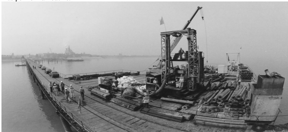
Figure 4: Steel trestle and drilling platform
