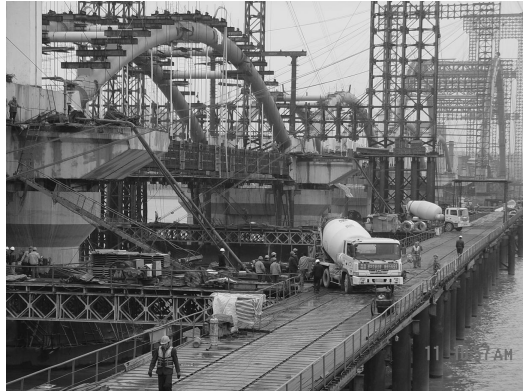
Figure 9: The concrete was pumped from both sides of the abut into steel pipe arch rib
