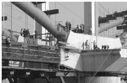
Figure 10: The workers were connecting the concrete duct
