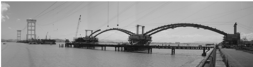
Figure 8: Full view of cable hoisting and installing system of Qiantangjiang 4th Bridge
