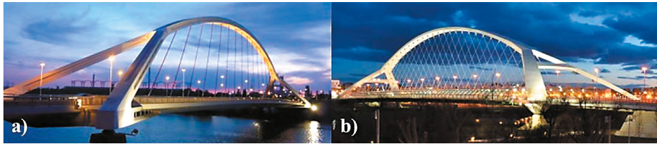
Fig. 8. a) Barqueta Bridge and b) Third Millennium Bridge.
