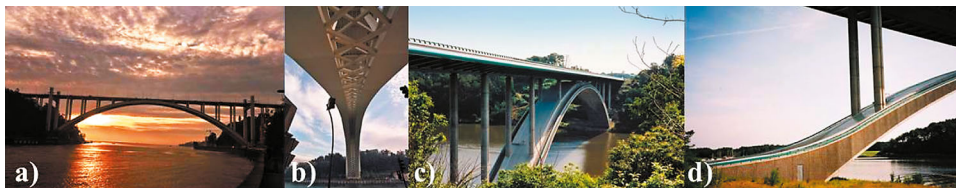
Fig. 4. a), b) Arrábida Bridge and c), d) Morbihan Bridge.
