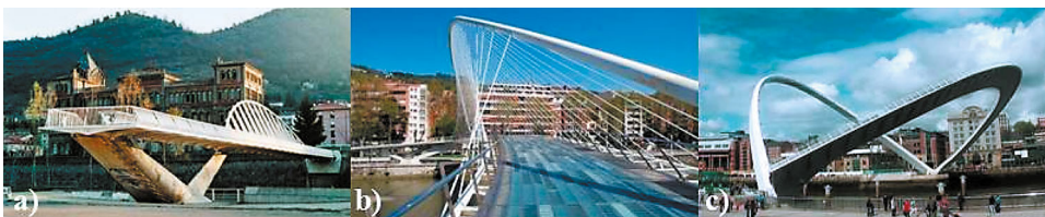
Fig. 10. a) La Devesa Bridge, b) Campo Volantin Bridge and c) Gateshead Millenium Bridge.
