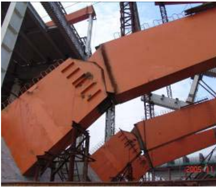
Figure 8 : The vertical swing hinge
