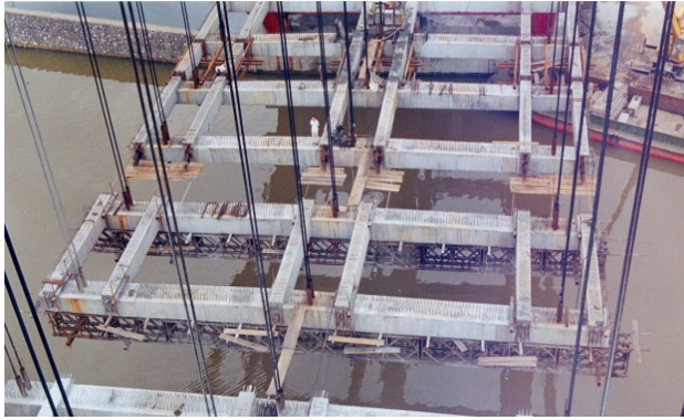
Fig. 10. Forming long lateral beam.
