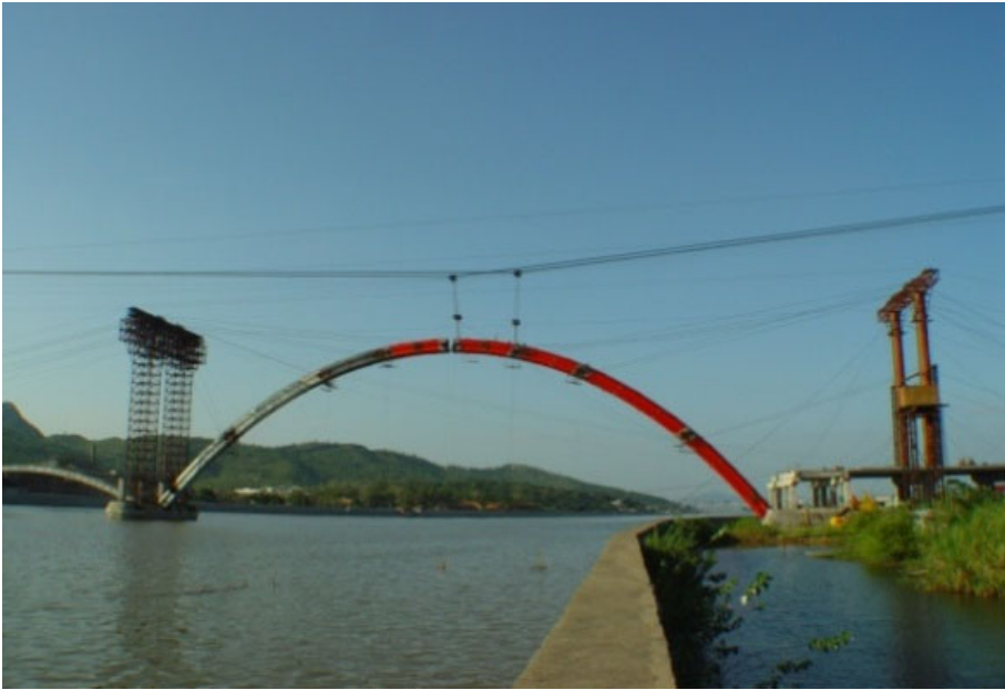
Fig. 4. Closure of single arch rib.
