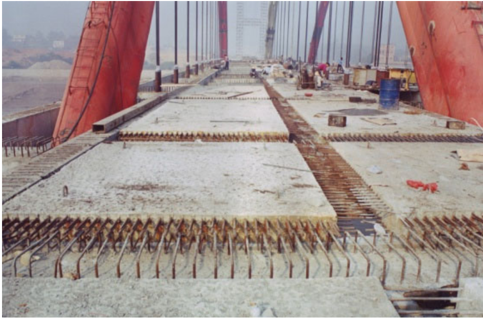
Fig. 13. Casting the joints of bridge deck.
