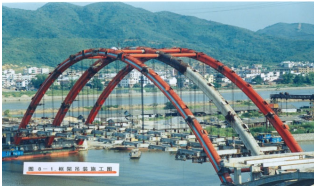
Fig. 8. Hoisting small frame.
