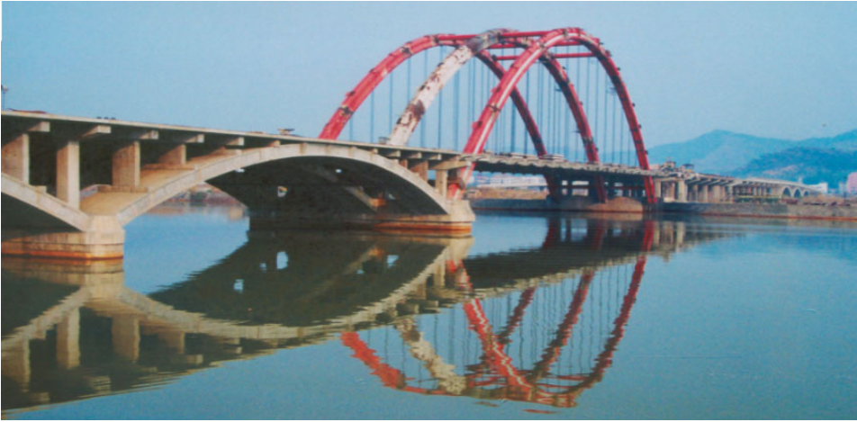
Fig. 1. Scenery of Baiwang bridge in Shaoguan in Guangdong.
