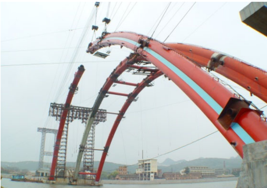
Fig. 5. Closure of three arch ribs.
