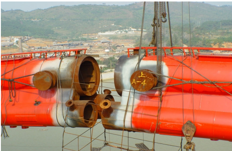
Fig.3. Middle joint of three-tube type.
