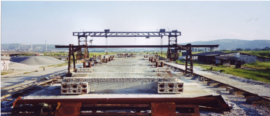
Fig. 7. Precasting rectangular small frame.
