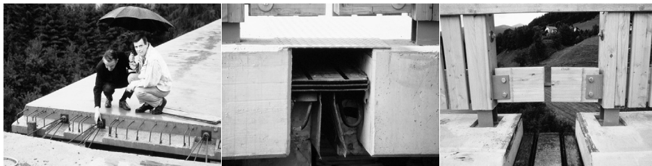
Figure 4 : Prestressed concrete slabs (left); Dilation in bridge center (middle); Dilation system of the waist rail (right).
