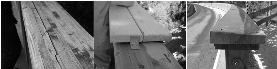
Figure 9 : Condition of the handrail in 2003 (left); Additional cover measures (middle, right).
