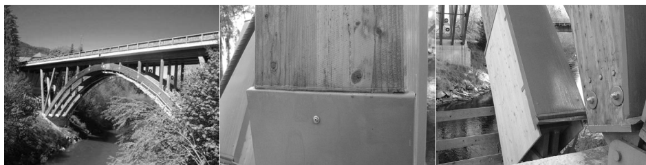
Figure 8 : Finished coating of the left bridge side (left); Renewed flexible seals (middle); Additional measure: encased arch bearing point (right).
