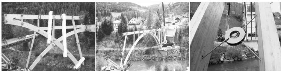
Figure 5 : Assembling of the main structure (left, middle); Threading of the connection brace (right).
