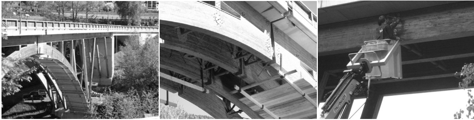
Figure 6 : Platform for the work at the main structure (left, middle); Joints: control of the firm fit (right).
