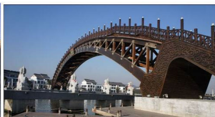
(b) Xujiang Bridge in China
