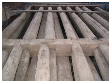
b) The mortise and tenon nodes.
