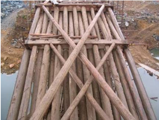
Fig. 9. The X-bracings.
