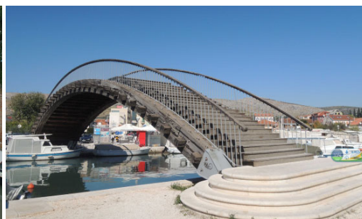
b) Timber rib arch bridge in Croatia
