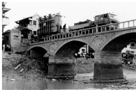
Figure 17: 50MVA main transformer past through the Jiang-kou Bridge.
