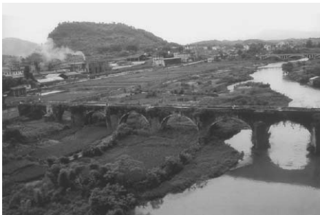
(a) Full view of the bridge.
