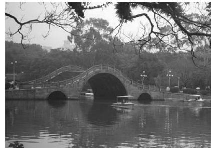
Figure 9: West lake park bridge.
