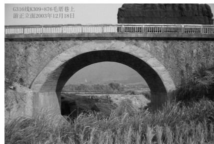
(b) After reinforcement
