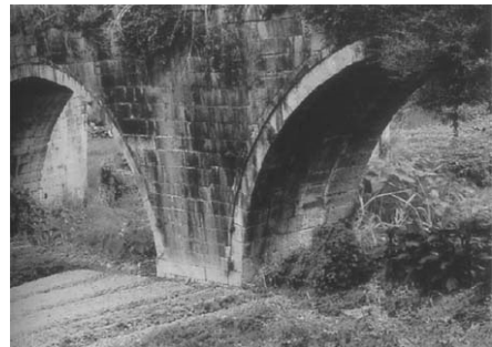
(b) Local view of the pier.
