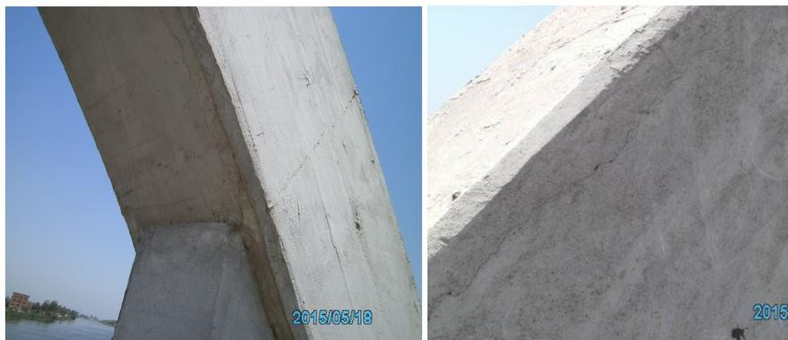
*Fig. 4. Non-structural cracks of the arch girders.*
