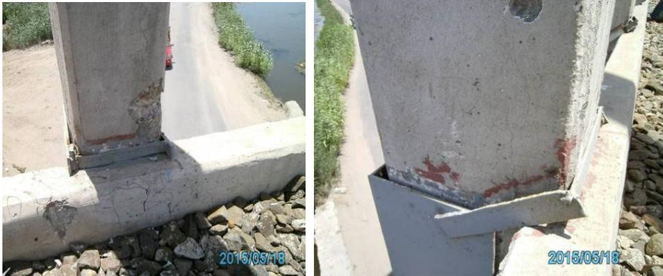
*Fig. 6. Damage of hangers of spans 1 and 5.*
