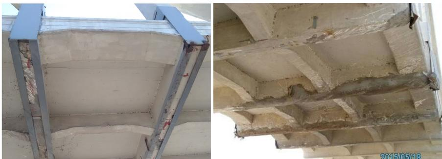
*Fig. 5. Damage of transverse beams of spans 1 and 5.*
