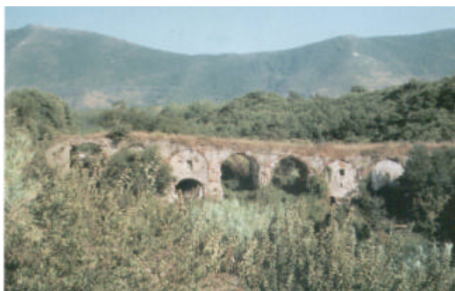
Figure 1. Ronaco viaduct-bridge in Sessa Aurunca.
