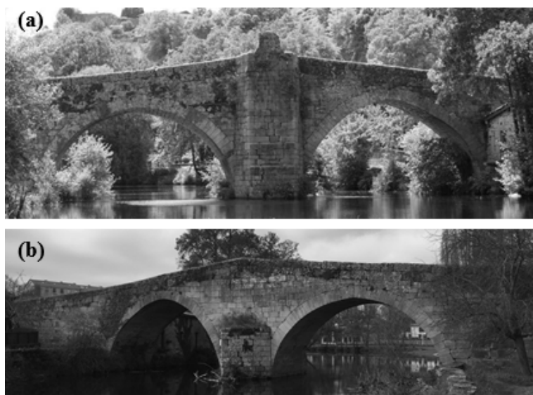
Fig. 1. General view of the Villanova bridge from (a) downstream side (b) upstream side.
