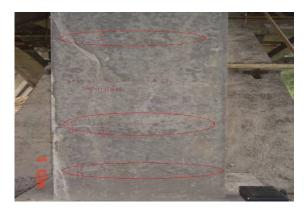
Figure 10 : horizontal cracks on pilars
