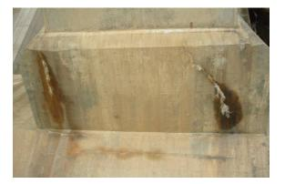
Figure 8 : cracks and water seeping on springing
