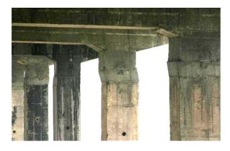
Figure 9 : pillars on the arch installed with error
