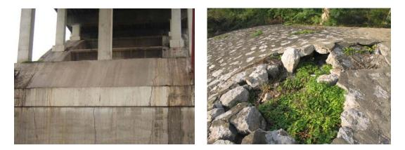
Figure 11: cracks and water seeping on skewback Figure 12: sink and crush on conical slope
