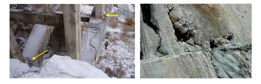
Figure 5 : Cracks and peeling of concrete on arch
