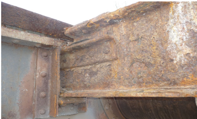
Fig. 7. Corrosion of longitudinal beam next to first crossbeam.
