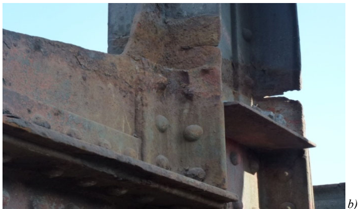
Fig. 6. a) Corrosion of supporting column and b) crack of hanger next to the crossbeam.
