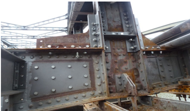
Fig. 9. The way of repair of hanger-cross beam connection and strengthening of the web of crossbeam.
