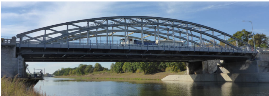
Fig. 11. Jagiellonian Old South bridge during the load test (10/01/2015).
