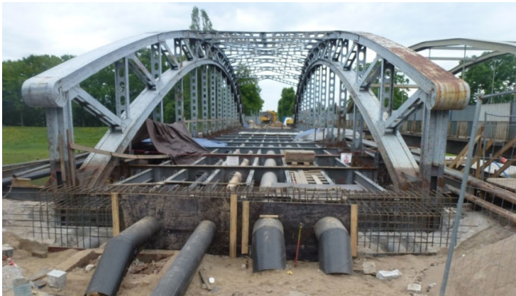
Fig 4. The reinforcement of the wall of the abutment.
