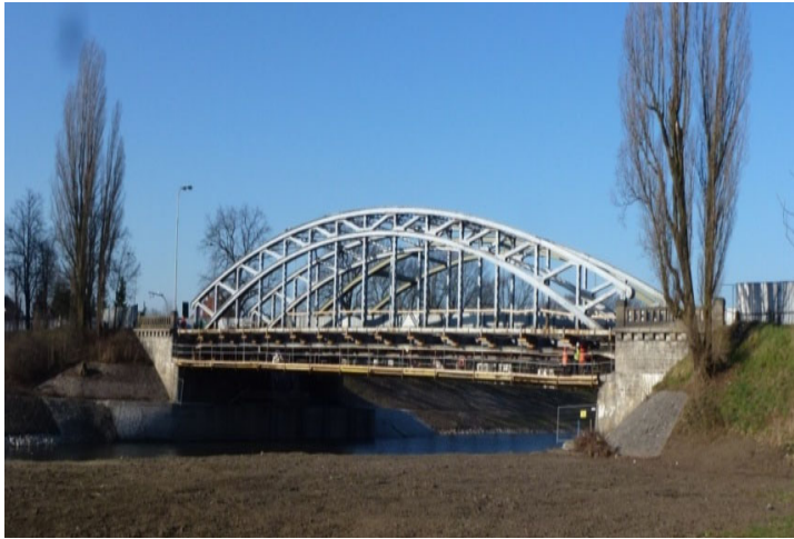
Fig. 3. A general view of the bridge during repair.
