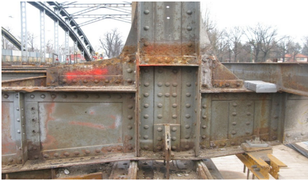
Fig. 8. Corrosion of crossbeam and hanger at midspan.
