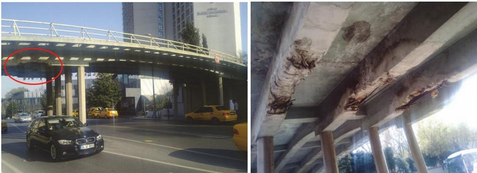
Figure 4: Old footbridge and its damages
