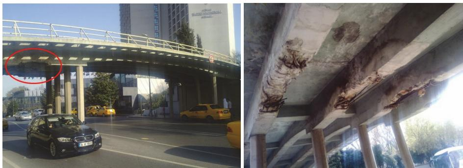
Figure 4: Old footbridge and its damages
