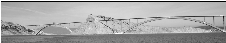
Figure 2: Krk bridges completed in 1980.
