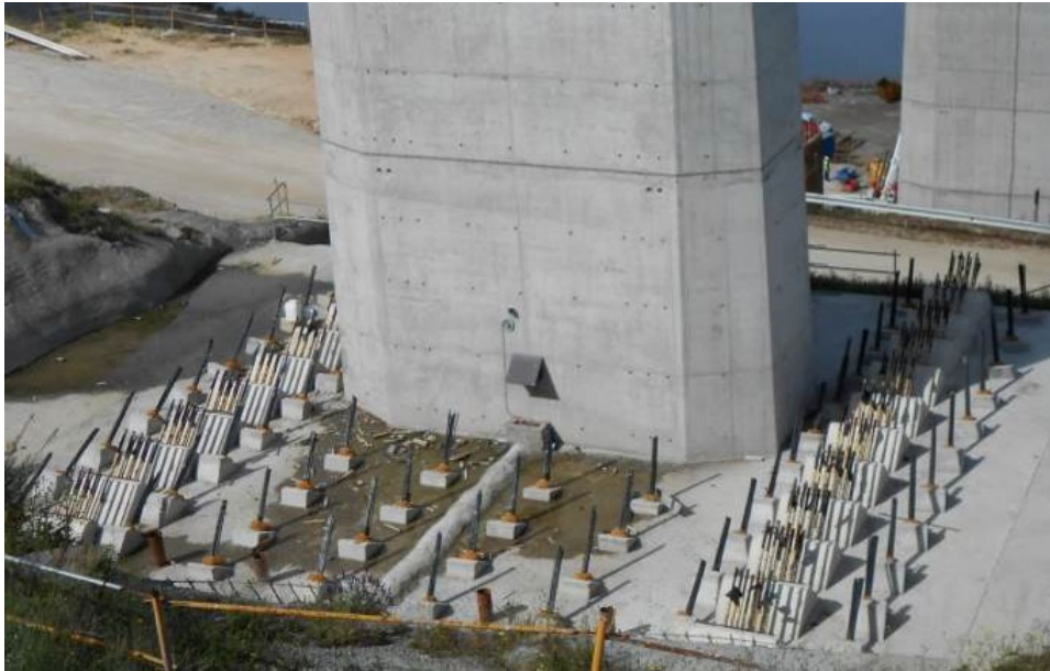
Fig. 7. View of one retaining foundation with anchorages for both bed-rock and stay cables.
