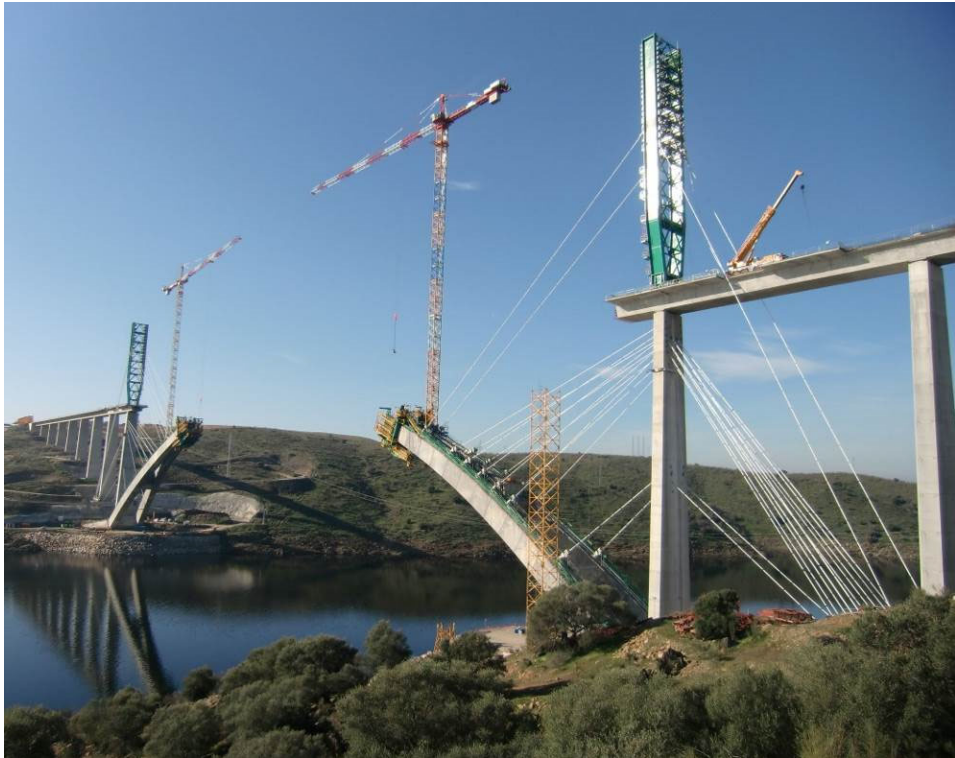
Fig. 3. Arch's cantilevered stage construction.
