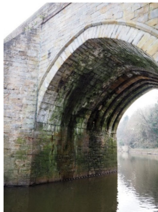
Fig. 7. Widened Elvet Bridge – photograph shows additional ribs.
