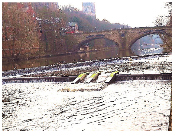
Fig. 4. Weir fixing the springing level of the bridge.
