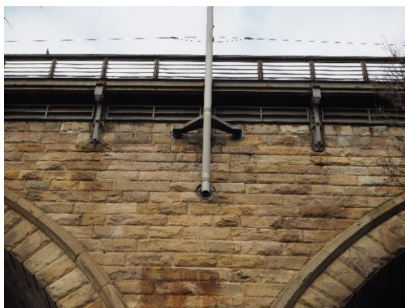
Fig. 12. Fixing of the Overhead Line Equipment to the Viaduct.
