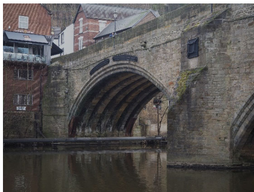
Fig. 5. Ribbed arches and through-ties of Framwellgate Bridge.
