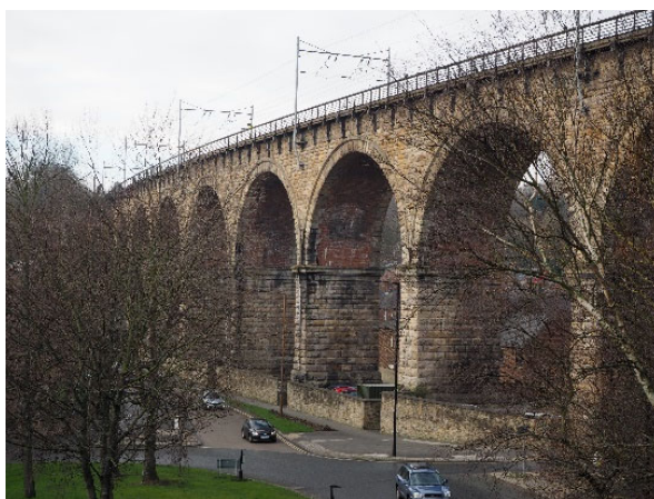
Fig. 11. Durham Viaduct in 2016.
