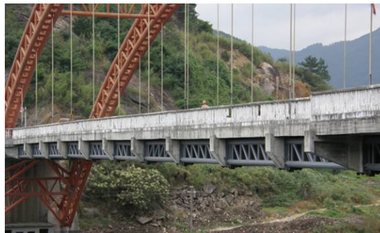
Figure 6 : Shitanxi Bridge (after strengthening)
