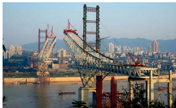
Figure 8 : Installation and Closure of Middle Span Arch
