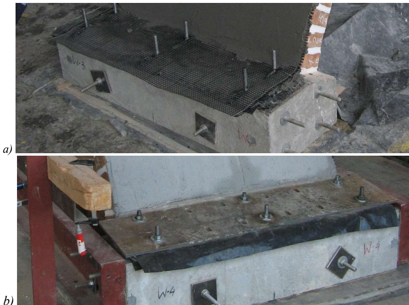
Fig. 3. a) Carbon fibre grid arrangement above the abutment – during application of the strengthening – arch VC-An. b) View of the strengthening's anchorage on the abutment of arch VC-An.
