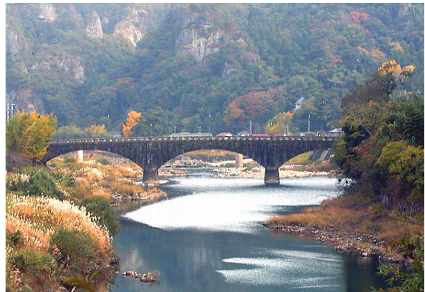
Figure 1: Rakanji Stone Arch Bridge
