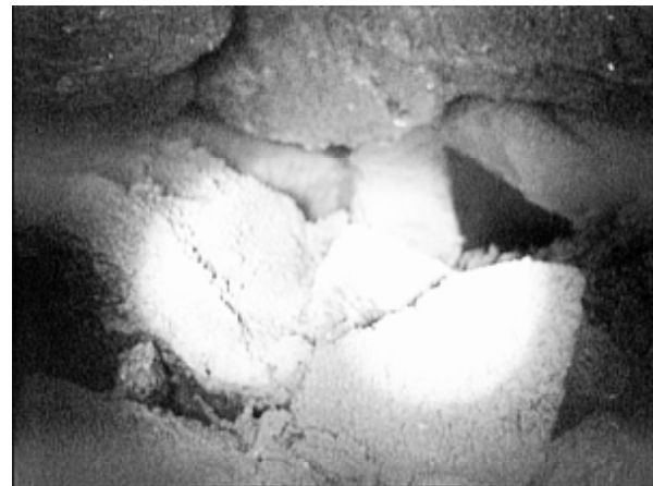
Figure 10: State of Stuffing Stones Observed by Fiberscope
