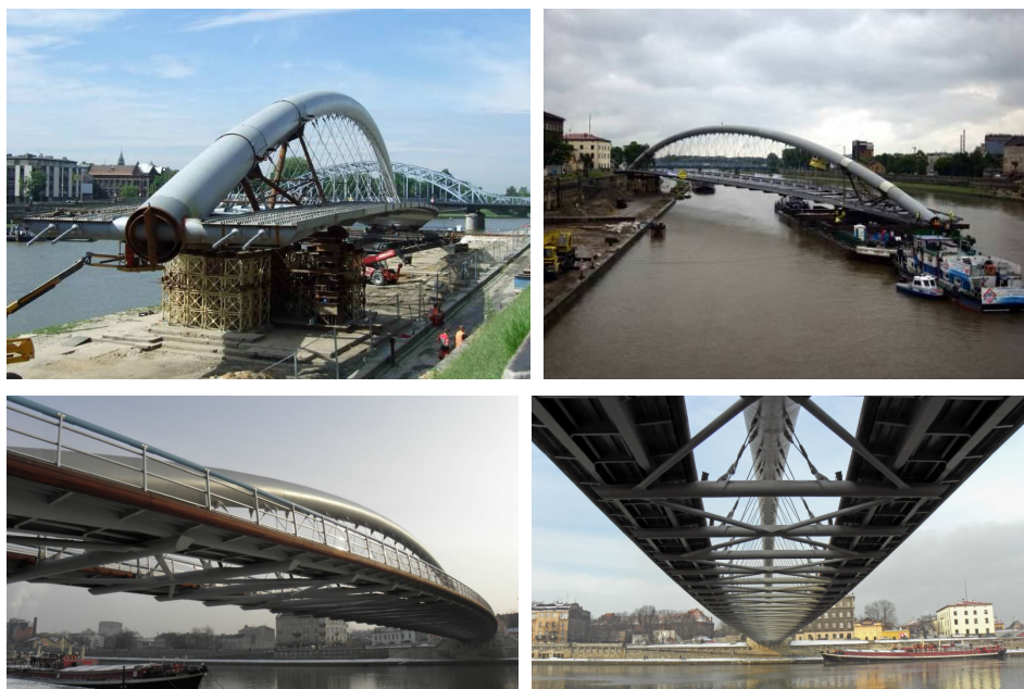
Fig. 6. Rotation of the arch span of the Father Bernatek Footbridge [6] and views of finished footbridge (photo: Ł. Chamów)
