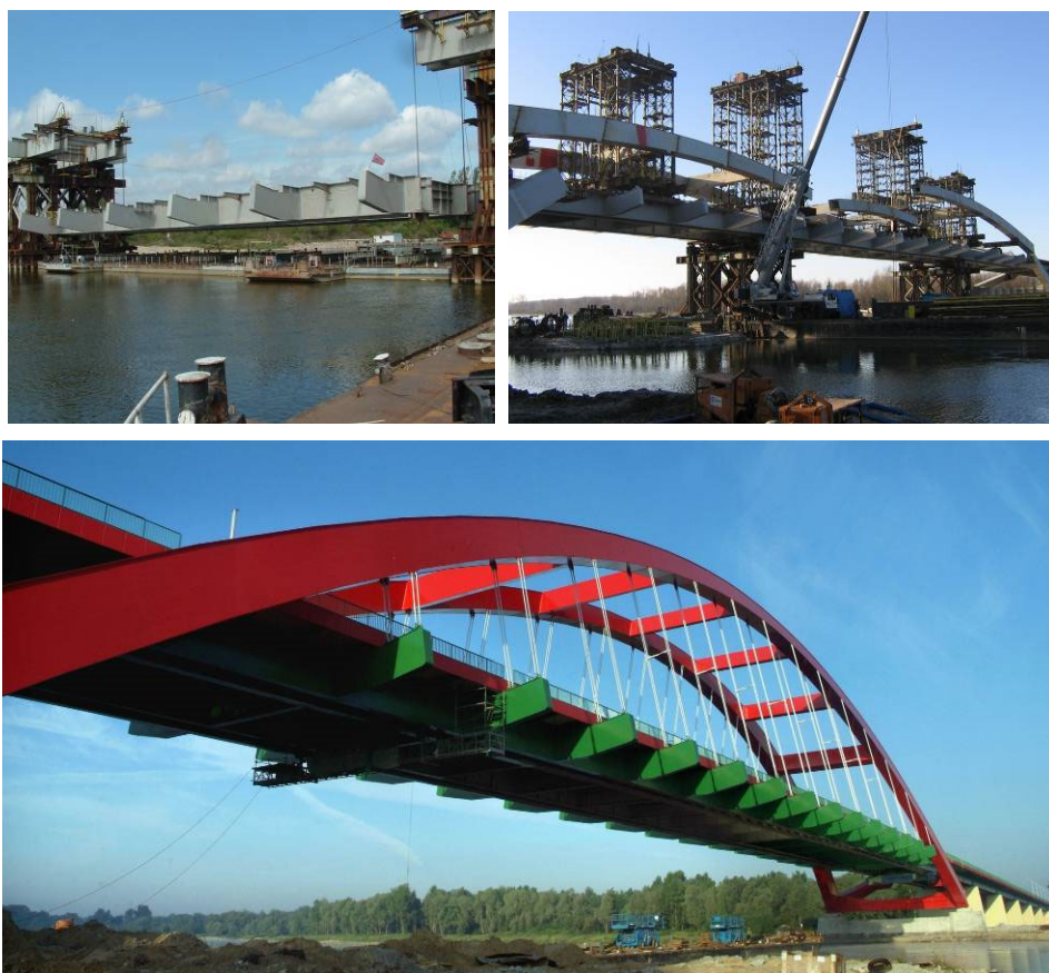
Fig. 2. Bridge in Puławy – main span construction [2] and view of completed bridge.
