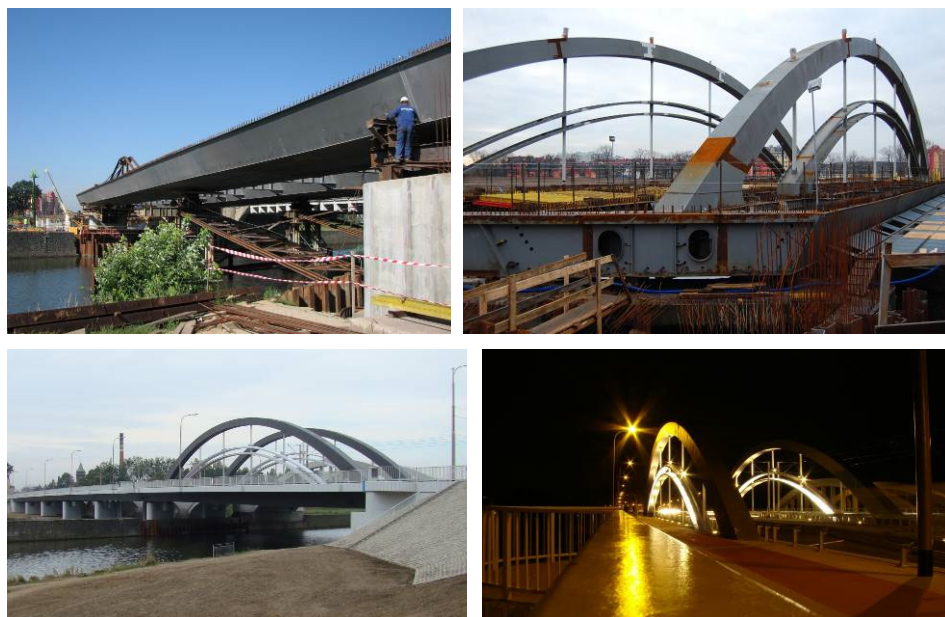
Fig. 5. Launching of the new Warszawski Bridge and views of finished structure.
