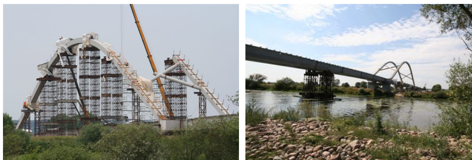
Fig. 4. Bridge in Gorzów Wielkopolski – assembly of arch girders and launching the bridge over the Warta River [4].
