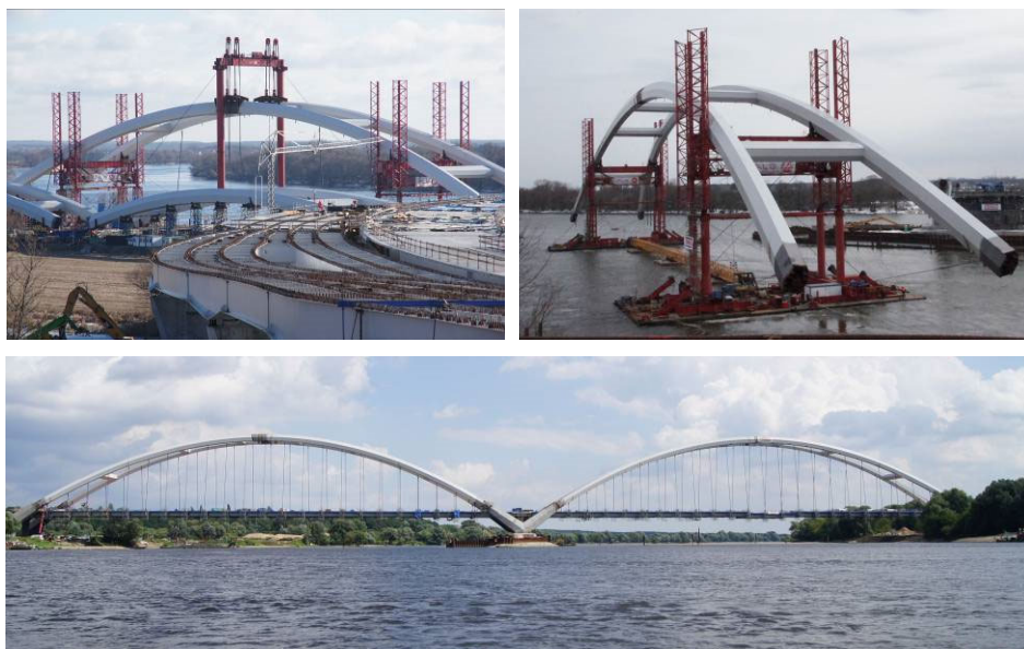
Fig. 7. Bridge in Toruń - assembly of steel arches using floating temporary supports (photo: K. Jędrzejewski, Strabag) and view of completed bridge.
