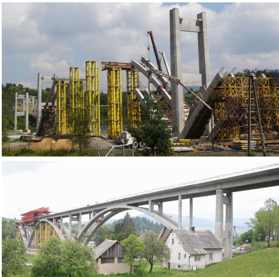
Fig. 3. Construction of the bridge in Milówka: assembly of precast arch elements (upper photo) [3], construction of the deck with use of a movable scaffolding (photo: PERI Polska).
