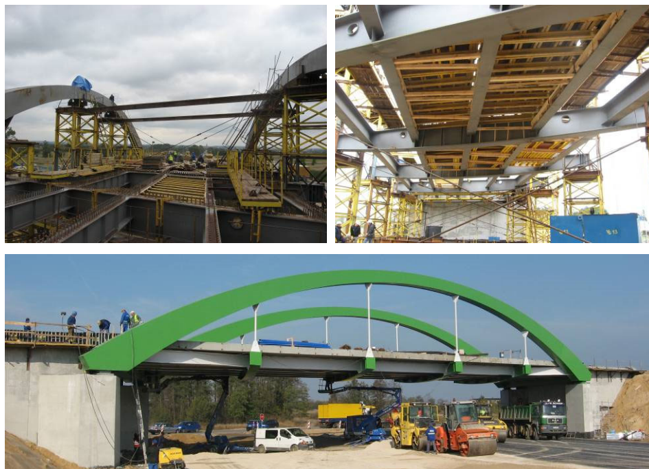
Fig. 1. Views of the viaduct in Stryków in different construction stages [1].
