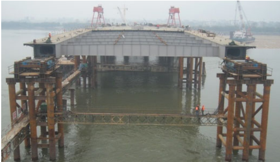
Fig. 12. Luozhou bridge under construction.
