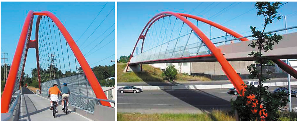
Fig. 16. McLoughlin Boulevard Pedestrian Bridge, Portland, Oregon, USA.
