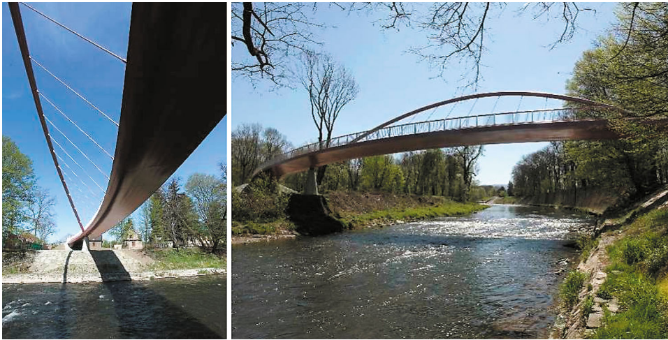
Fig. 21. Pedestrian bridge across the border River Olse, Czech and Polish Tesin.
