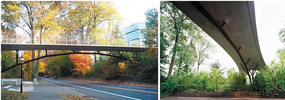
Fig. 8. Streicker Pedestrian Bridge, Princeton, New Jersey, USA.
