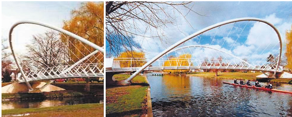
Fig. 18. Butterfly Bridge over the River Great Ouse, Bedford, UK.
