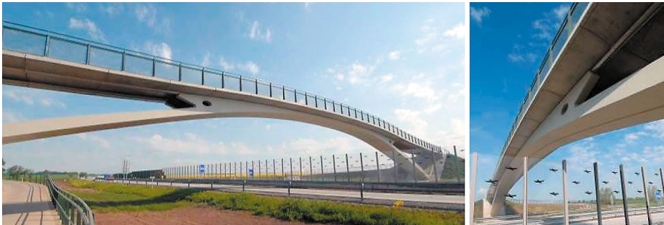
Fig. 28. Pedestrian Bridge across the Expressway R35 near a city of Olomouc, Czech Republic.
