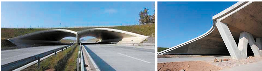
Fig. 6. Bridges across the Motorway D1, Czech Republic.
