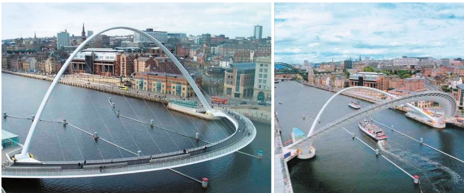
Fig. 20. Gateshead Millennium Bridge spanning the River Tyne, Newcastle, UK.
