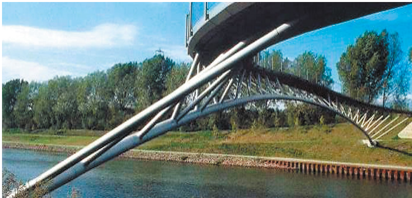
Fig. 9. Ripshorst Pedestrian Bridge, Germany.
