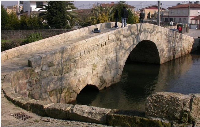
Fig. 3. General view of the Lazaro Bridge.
