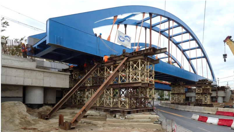
Fig. 9. Span no. 2 during the transverse slide over on support PS-L into its final position on track no. 2 of Line No. 271.
