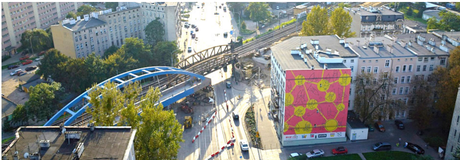
Fig. 7. Span no.1 during the launching process over Grabiszyńska Street (source: fotopolska.eu).
