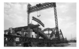
Figure 10: Temperay Bridge and Gantry Crane
