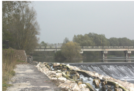
Figure 3: A section of the bridge surrounded by the vegetation
