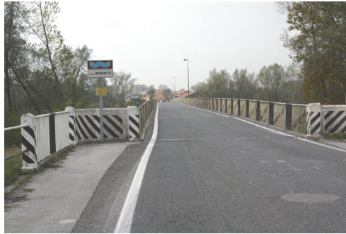
Figure 1: The “bottleneck” on the bridge
