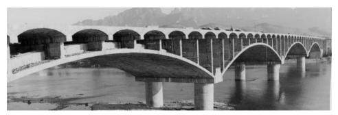
Fig. 5. Guanyin Bridge with coping of buttress, spandrel arch ring cantilevered  $2 \times 1$  m each,  $(2\Phi 3.5 \text{ m hollow pier})$ .
