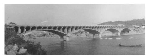
a) Lusiwan Bridge with cantilevered PRC beam for the deck structure, (2 $\Phi$ 3m-2 $\Phi$ 5m digging pile)
