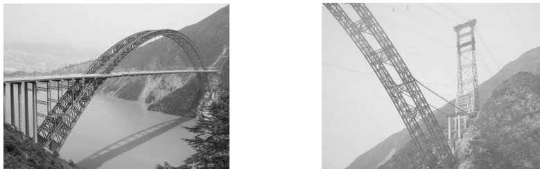
Figure 13 : Wushan Yangtze River Bridge
