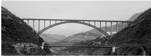
Figure 12: Fengjie Meixihe Bridge
