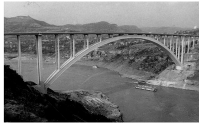
Figure 2 : Wanxian Yangtze River Bridge
