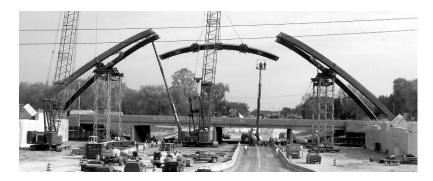
Figure 15: Erection of center rib with temporary towers
