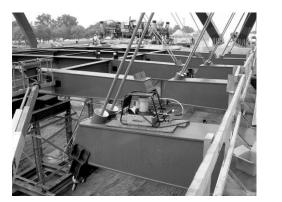
Figure 11: Hanger assembly - two strands
