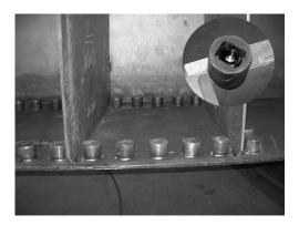
Figure 13 : Nut cover cup welded to arch rib
