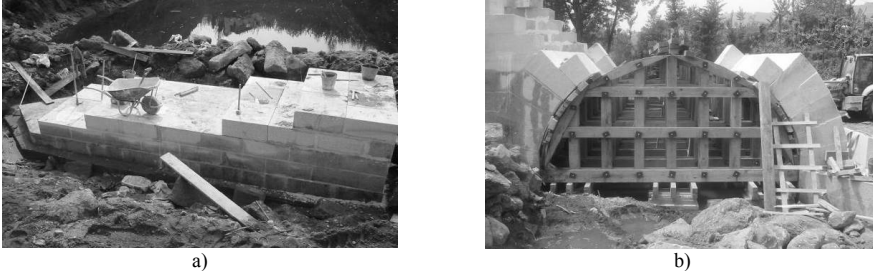
Figure 3 : Vila Fria bridge structure – (a) piers and (b) arches
