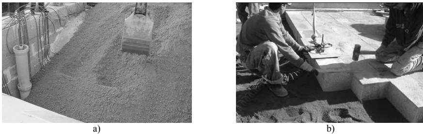
Figure 4 : Vila Fria bridge structure – (a) backfill material and (b) granite stone pavement
