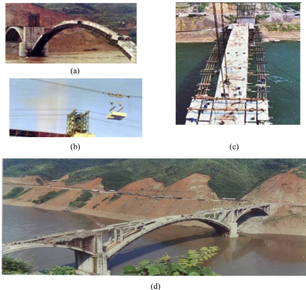
Figure 5 : 135m box arch construction(a)Erection of No.2 box blocks after No.1 boxes, (b)Erecting box block by cable over the tower top, (c)Erection of No.3 and No.4 connection of after connection of middle three boxes, (d)Erection of columns and hollow slabs on the top of arch
