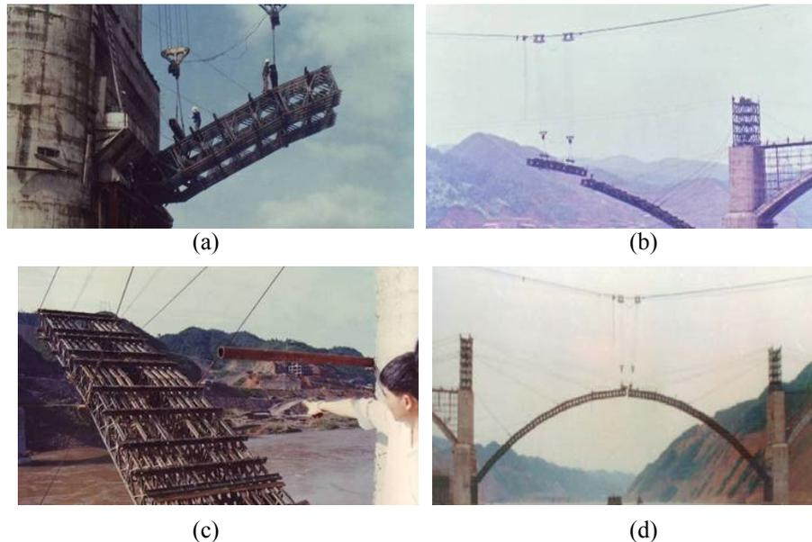
Figure 4 : Cable-stayed Bailey steel arch construction installation(a) Section A Steel arch construction installation, (b)Section C steel arch construction installation, (c) Midspan steel arch construction hanging, (d) Period before 133m middle-part connection
