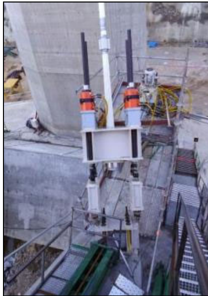
Fig. 14. Cable stay stressed.
