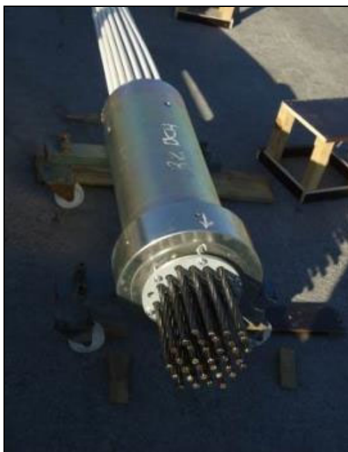
Fig. 10. Nut Head anchor assembly.
