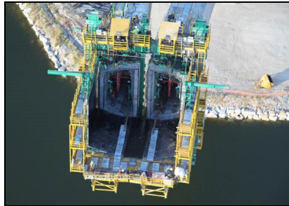
Fig. 8. Form travellers before union.
