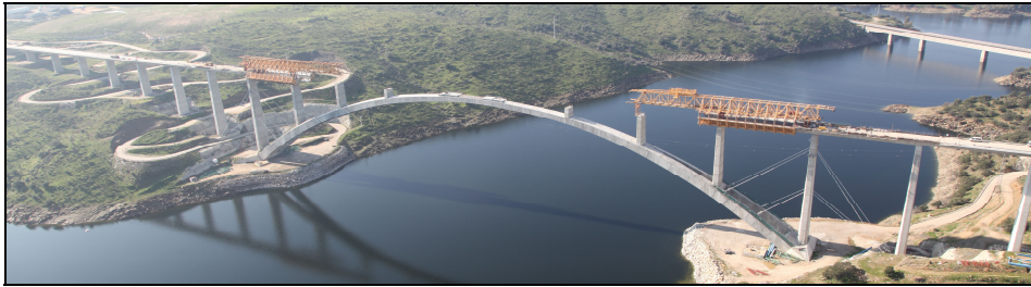
Fig. 16. Almonte Viaduct Current State.
