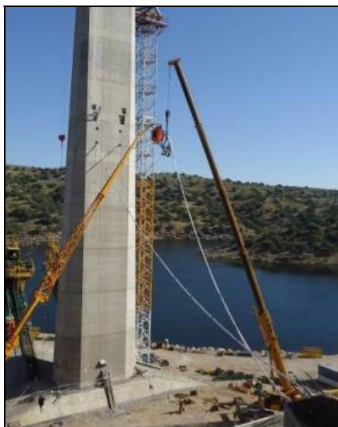
Fig. 11. Cable stay mounting.
