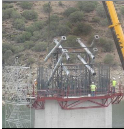
Fig. 5. Lower tubular structure.
