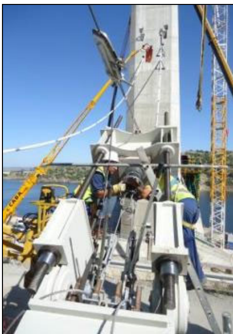
Fig. 13. Anchor head assembly.
