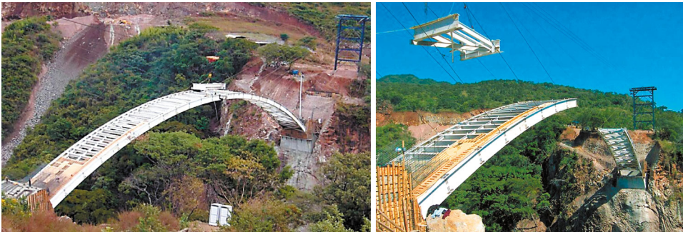
Fig. 5. Segments transporting and fixing (left) and Closing segment (right).
