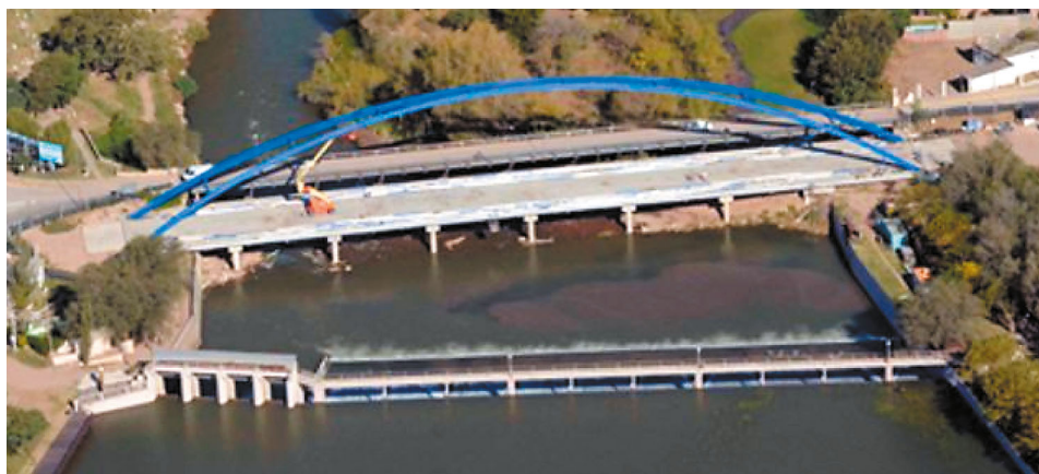
Fig. 18. Deck falsework and arches ready to start cable tensioning.
