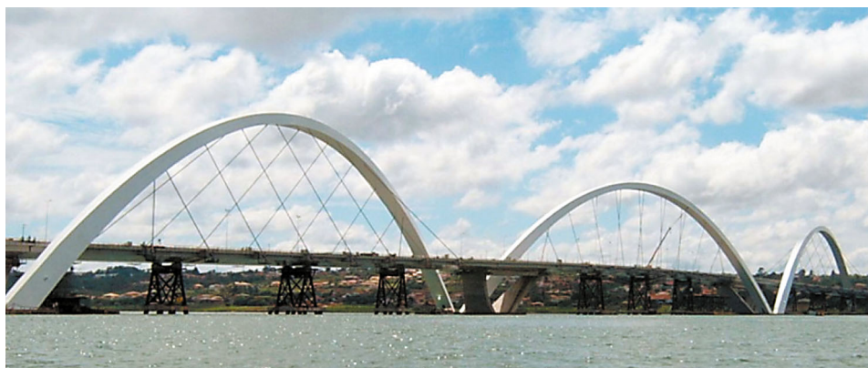
Fig. 12. The three arches, Clubs, Central, and Shis, supported on columns P5 to P8 (always from left to right).
