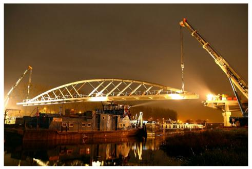
Fig. 7. Erection of the main span (photo: Ryszard Bugaj).
