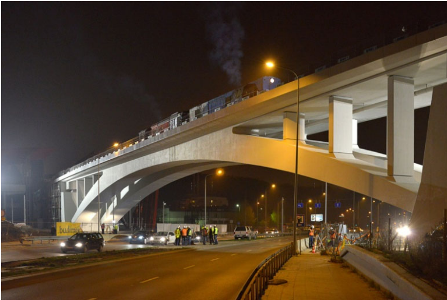
Fig. 7. Test load (photo – archive of PG).
