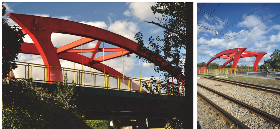
Figure 2: Views of the “shark’s fin” viaduct in Bydgoszcz (photos: K. Janikowska)
