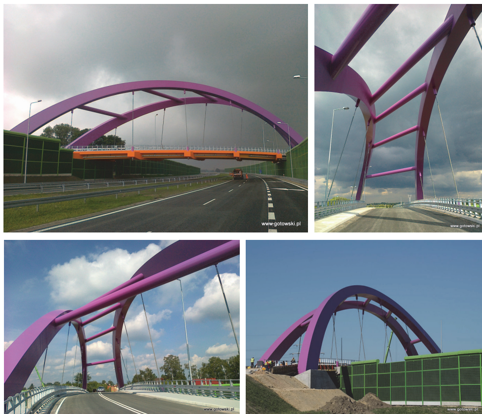
Figure 5: Views of the “crooked” viaduct near Pabianice (photos: www.gotowski.pl )
