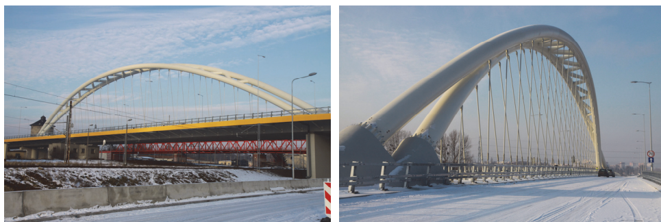
Figure 3: Views of the viaduct in Gdańsk under construction (photos: K. Topolewicz)
