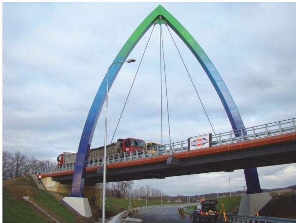
Figure 7: View of the viaduct in the Klucz interchange
