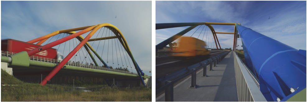
Figure 6: The "rainbow" viaduct over the A2 motorway (photos: K. Janikowska)
