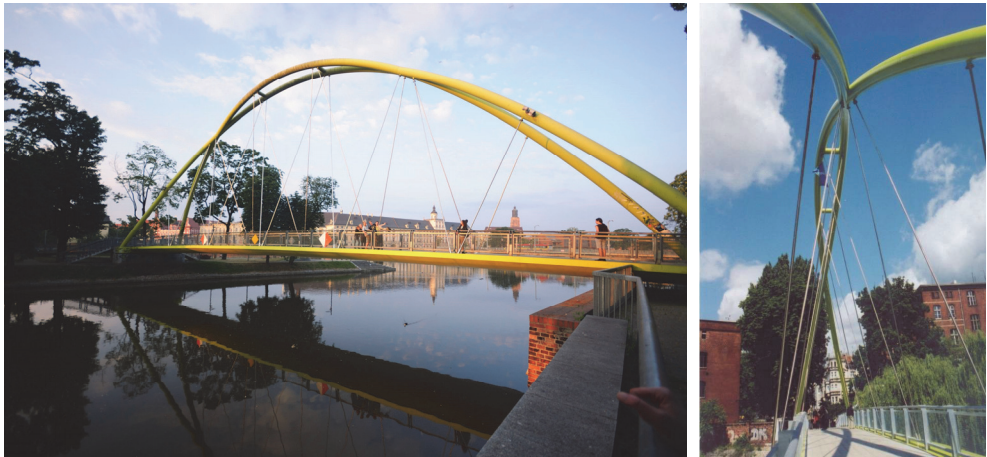
Figure 1: Views of the Ślódowa Footbridge in Wrocław
