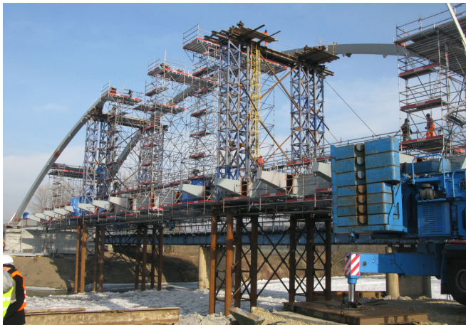
Fig. 8. Bridge erection – stage of arches assembling. Temporary supports and towers.
