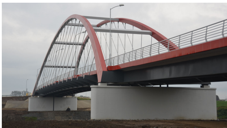
Fig. 7. General view on new-build bridge from level of terrain.
