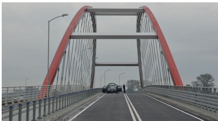
Fig. 6. General view on new-build bridge from level of a surface.
