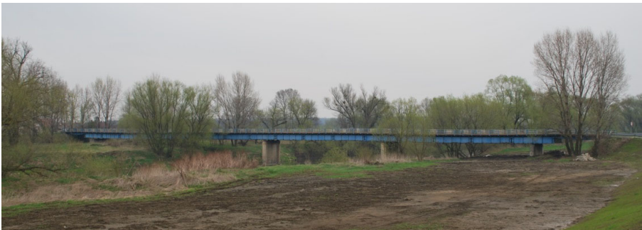
Fig. 1. General view on temporary bridge from the left bank of the Odra river.
