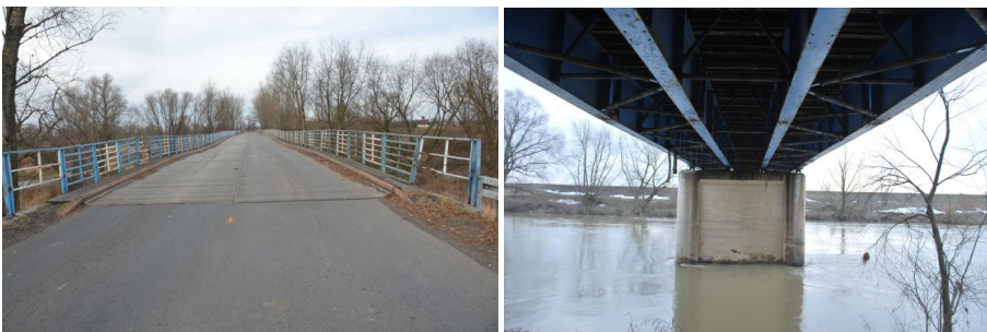
Fig. 2. General view on temporary bridge from surface layer level (on the left) and from the bottom side (on the right).
