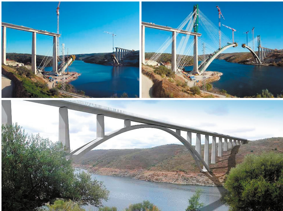
Fig. 17. Bridge over River Almonte, at Alcântara Reservoir (finished in 2016): construction sequence and rendering of the final bridge.
