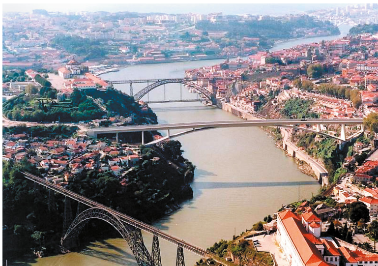
Fig. 20. Aerial view of Maria Pia, Infant Dom Henrique (built in 2003) and Luiz I Bridges.
