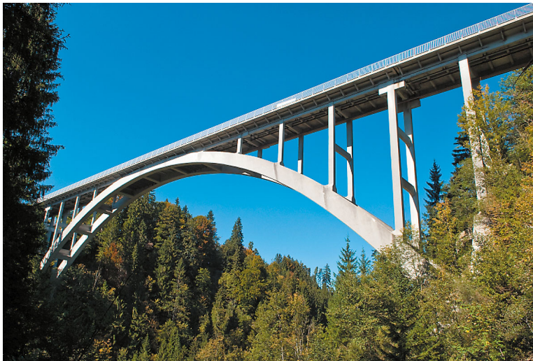
Fig. 9. Echelsbach Bridge over River Ammer – Germany (HaTe photo), 130 m span, designed by Heinrich Spangenberg and built in 1929.
