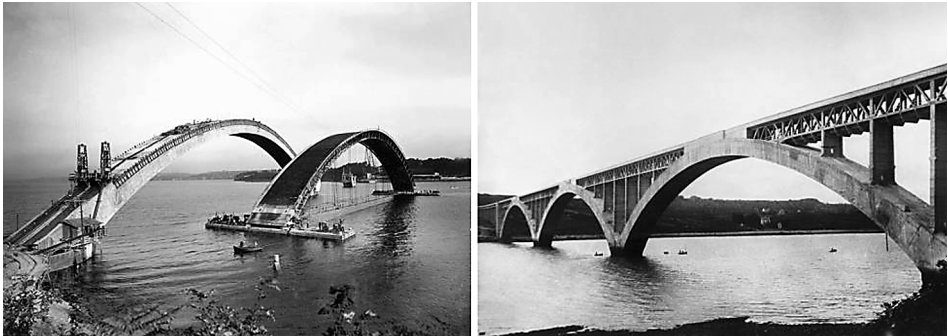
Fig. 4. Albert Louppe Bridge – France (3 spans of 186 m, built in 1930).
