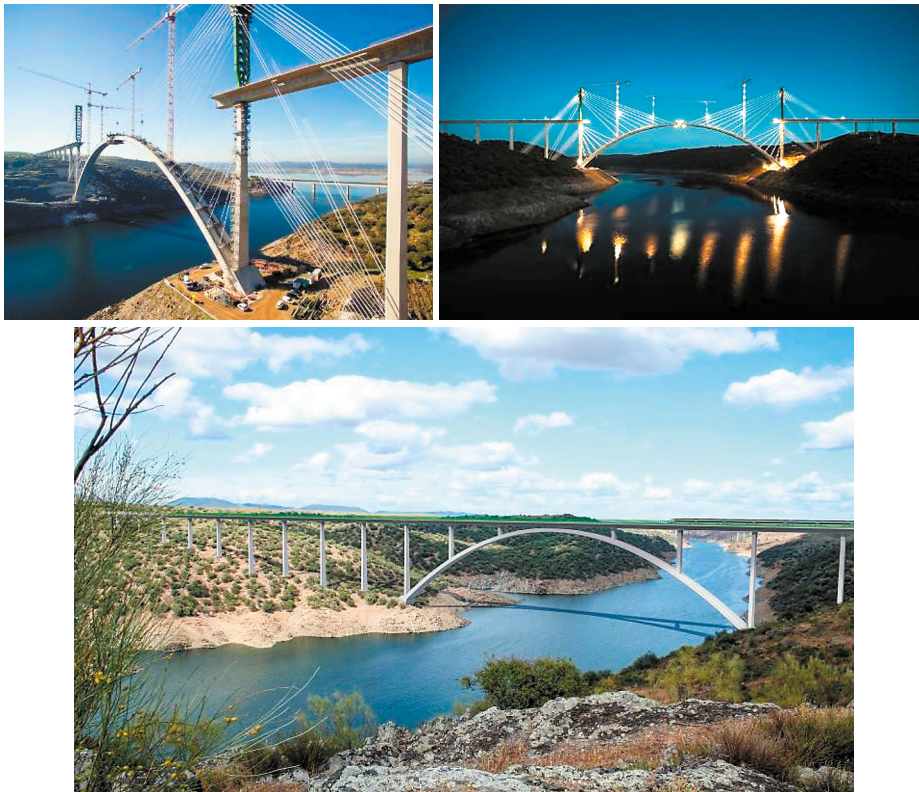
Fig. 16. Bridge over River Tagus, at Alcântara Reservoir (to be finished in 2016): construction sequence and rendering of the final bridge.
