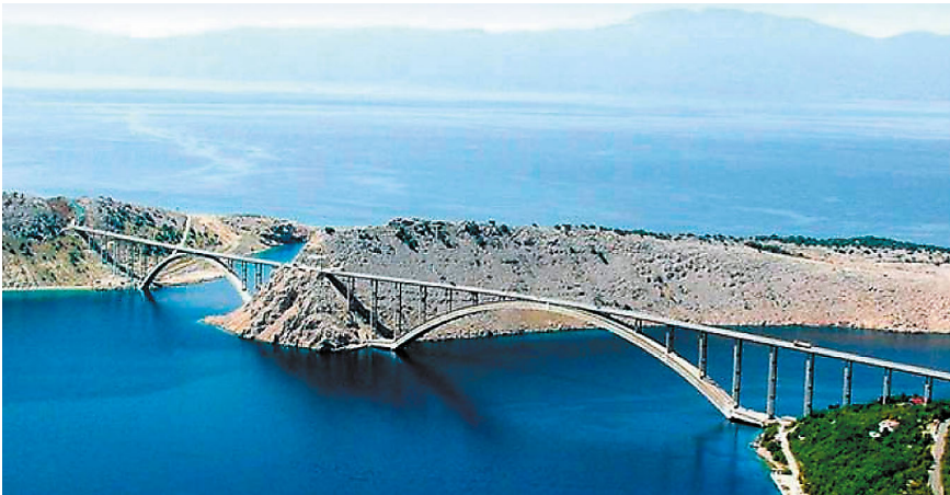
Fig. 14. Krk Bridges – Croatia.
