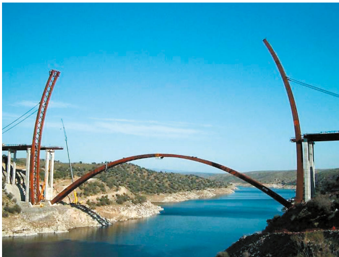
Fig. 13. Arcos de Alconéтар Bridge – Spain, designed by J A Llobart, J Revoltós and S Wörner, and built in 2006.
