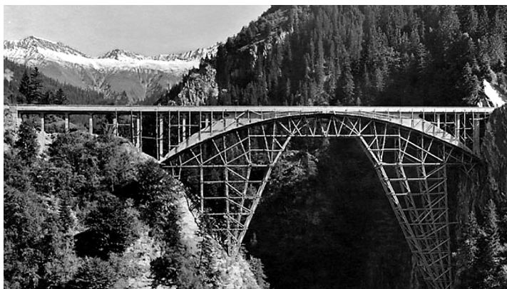
Fig. 3. Salginatobel Bridge – Switzerland, 90 m span, designed by Robert Maillart and built in 1930.
