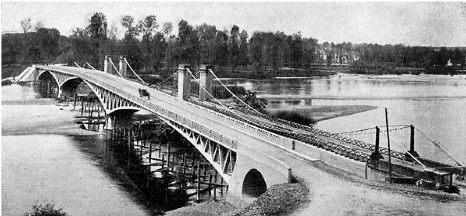
Fig. 1. Veudre-sur-Allier Bridge (72.50 m central span, built in 1912).
