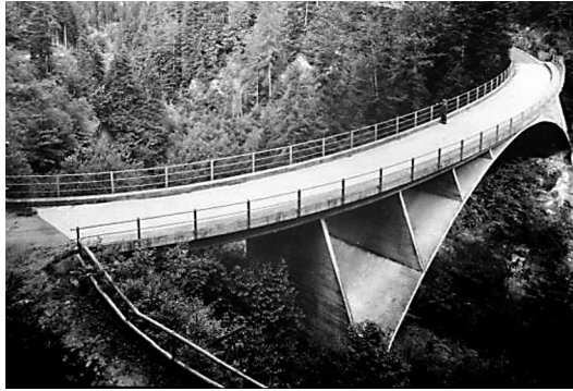
Fig. 18. Schwandbach Bridge – Switzerland (37 m span, built in 1933).
