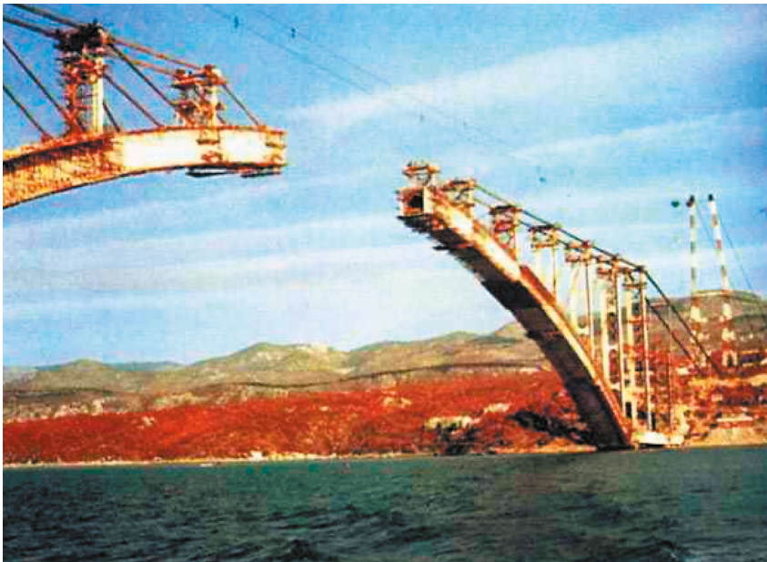
Fig. 15. Krk East Bridge under construction.
