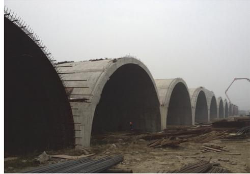
Figure 3: Arch rings were finished
