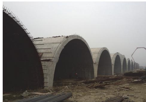
Figure 3: Arch rings were finished
