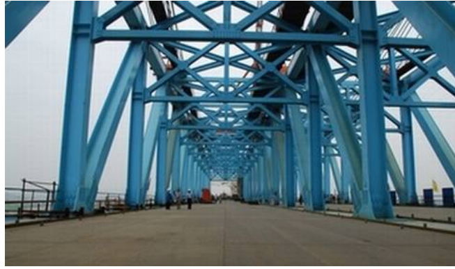
Figure 7 : The truss connections in Dashengguan Bridge
