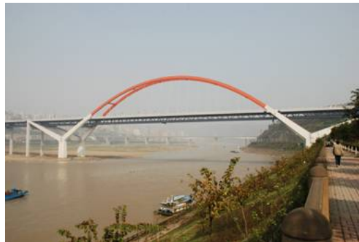
Figure 3 : Caiyuanba Yantze River Bridge in Chongqing
