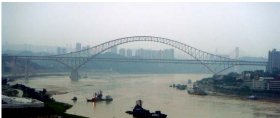
Figure 5 : Chaotianmen Bridge in Chongqing
