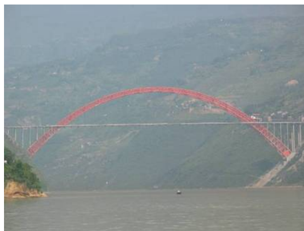
Figure 13 : Wushan Yangtze River Bridge
