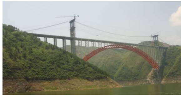
Figure 6 : Daninghe Bridge under construction
