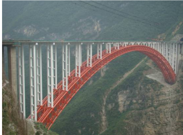
Figure 14 : Zhejinhe Bridge near completed
