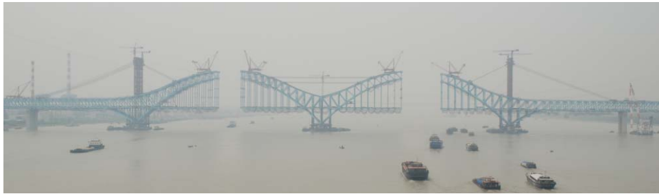
Figure 8 : Construction of Dashengguan Bridge
