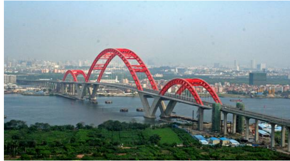
Figure 4 : Xinguang Bridge in Guangzhou
