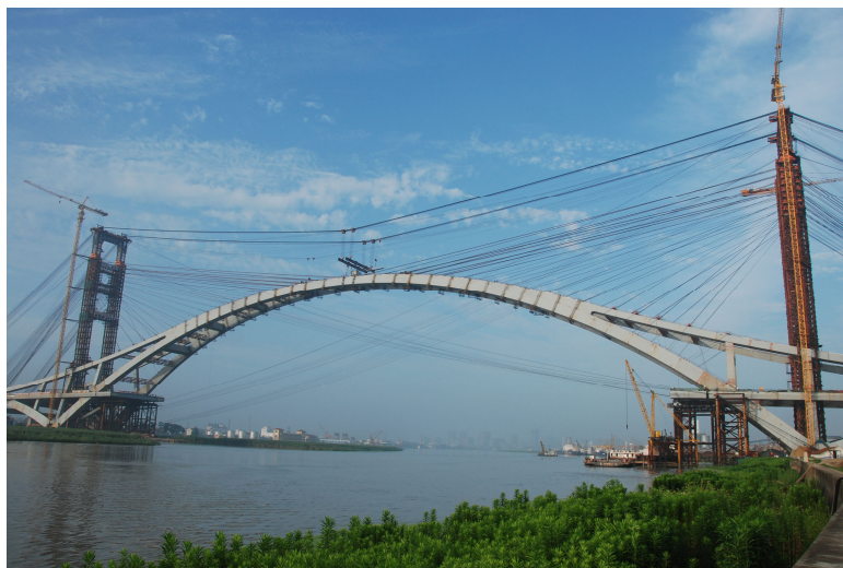
Fig. 8. Closure of the mid-span rib.
