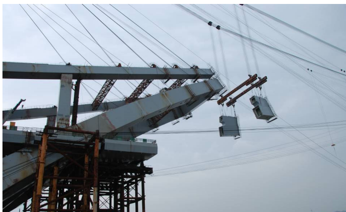
Fig.6. Flexible connection between the upper rib and the low rib.
