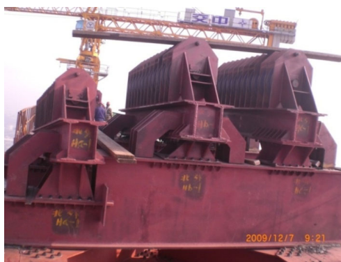
Fig. 3. Self-balanced cable saddle.
