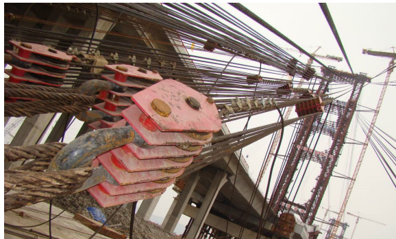
Fig. 5. Adjusting device of the main cable.
